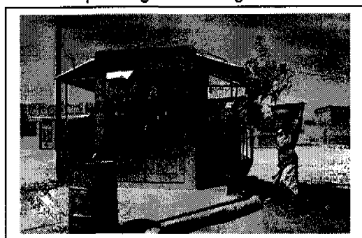
Photo 3 : PEA with electrical energy
