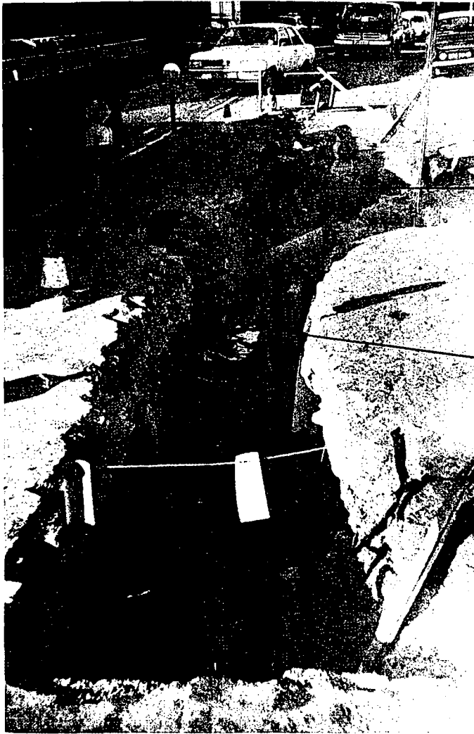
Figure 4. Thermoplastic pipe insertion technique. General view of excavation showing lead-in trench
