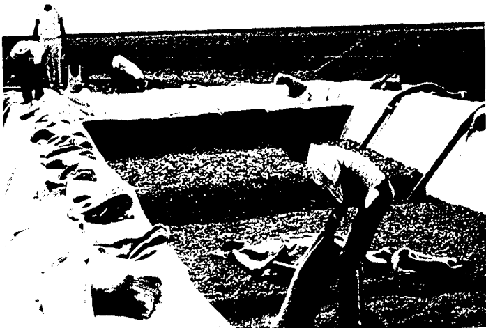
Fig. 47 Filling the HRF with filter material (pictures by the Swiss Disaster Relief Unit)
