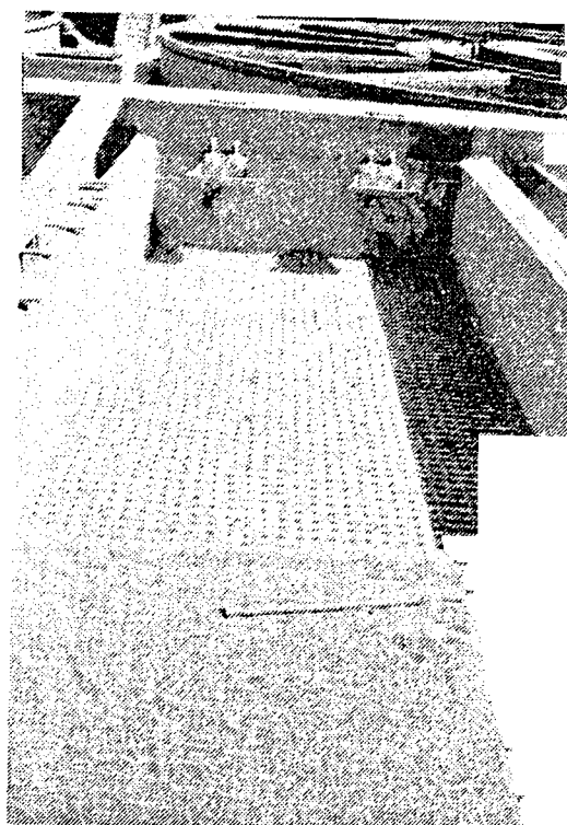
Fig. 4.32 Construction of false bottom and strainer underdrainage system.
