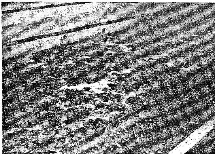
Fig. 3.2 Backwashing of a rapid filter.
