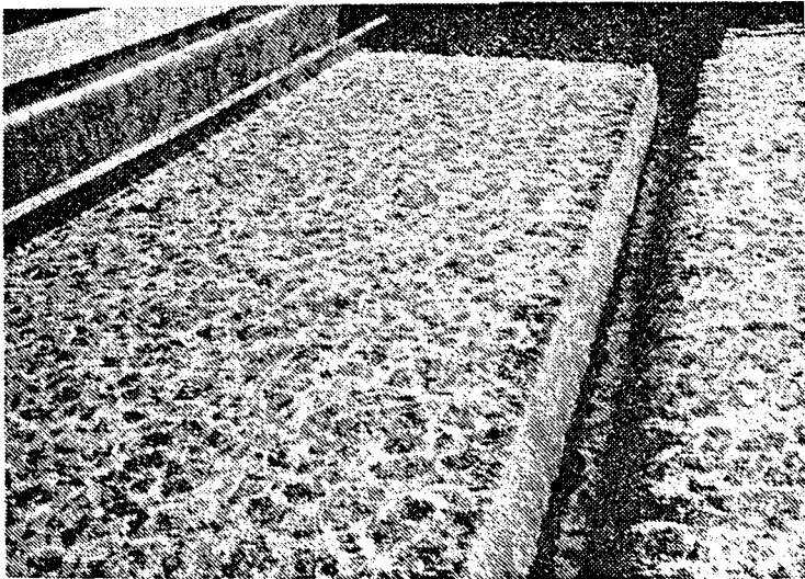
Fig. 3.33 Air wash combined with water wash.
