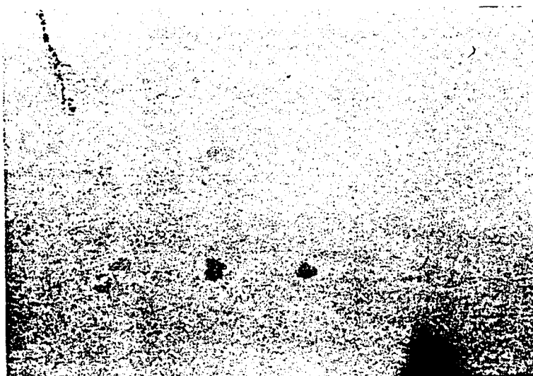
Fig. 4.23 Black spots on filterbed surface
