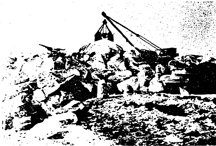
Fig. 2.7 Clearing away the ice at the Weesperkarspel plant for Amsterdam water supply
