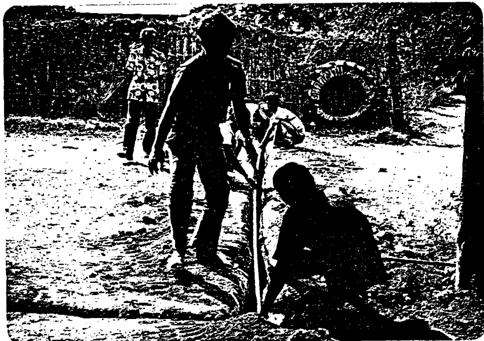
Fig. 39 Villagers participating in laying pipe line under closed attention of the village headman at Ban Thadindam, Lopburi Province.
