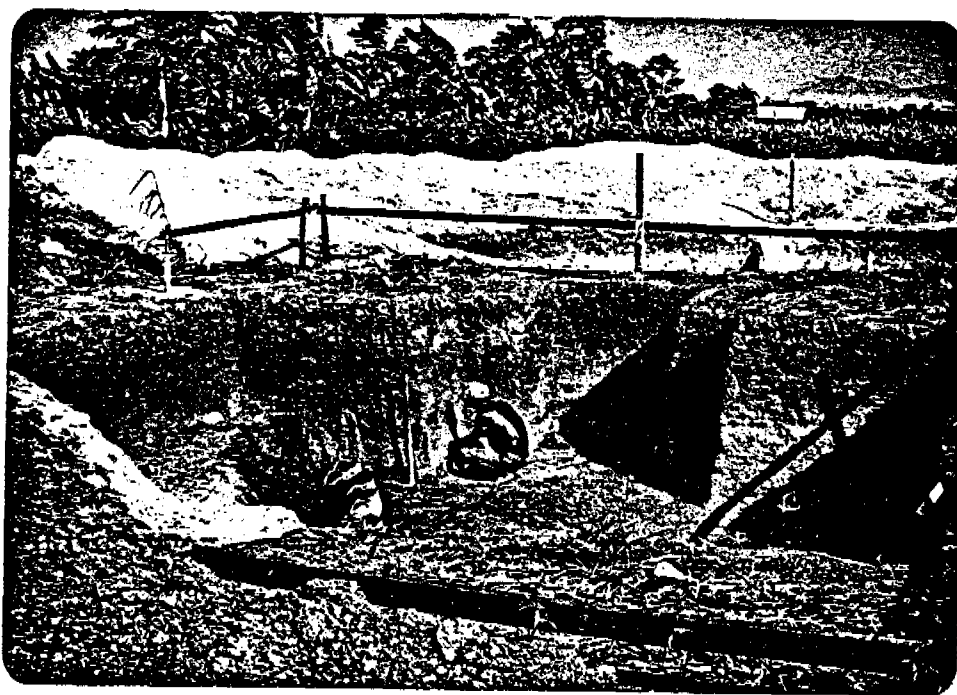
Fig. 25 Excavating the soil into the slow sand filter shape at Ban Thadindam, Lopburi Province.
