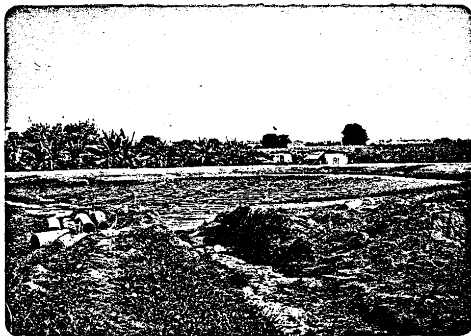
Fig. 23 View of a trough dug to convey water from the dam into the holding pond at Ban Thadingam, Lopburi Province.
