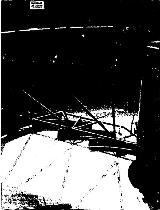
Fig. 3-63 Rotating sludge scraper suspended from revolving bridge.
