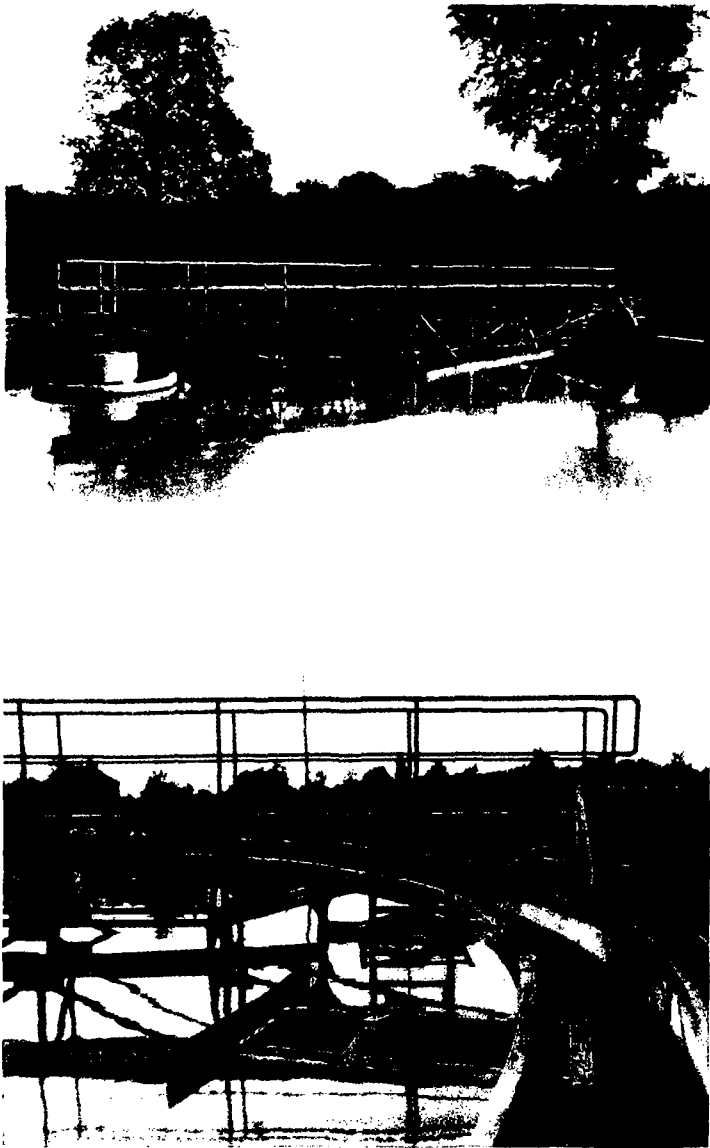
Fig. 3-69 Skimming in circular horizontal flow settling tanks.
