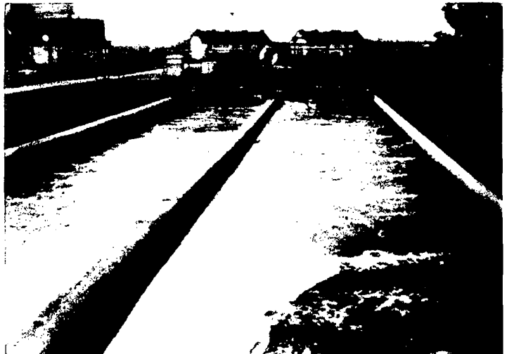
Fig. 5-15 Aerated grit chamber.
