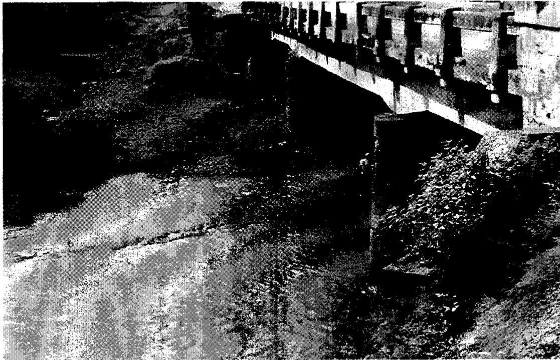
No. 2 Bridge on the Costal Highway (CA-2) over the El Rosario River.
