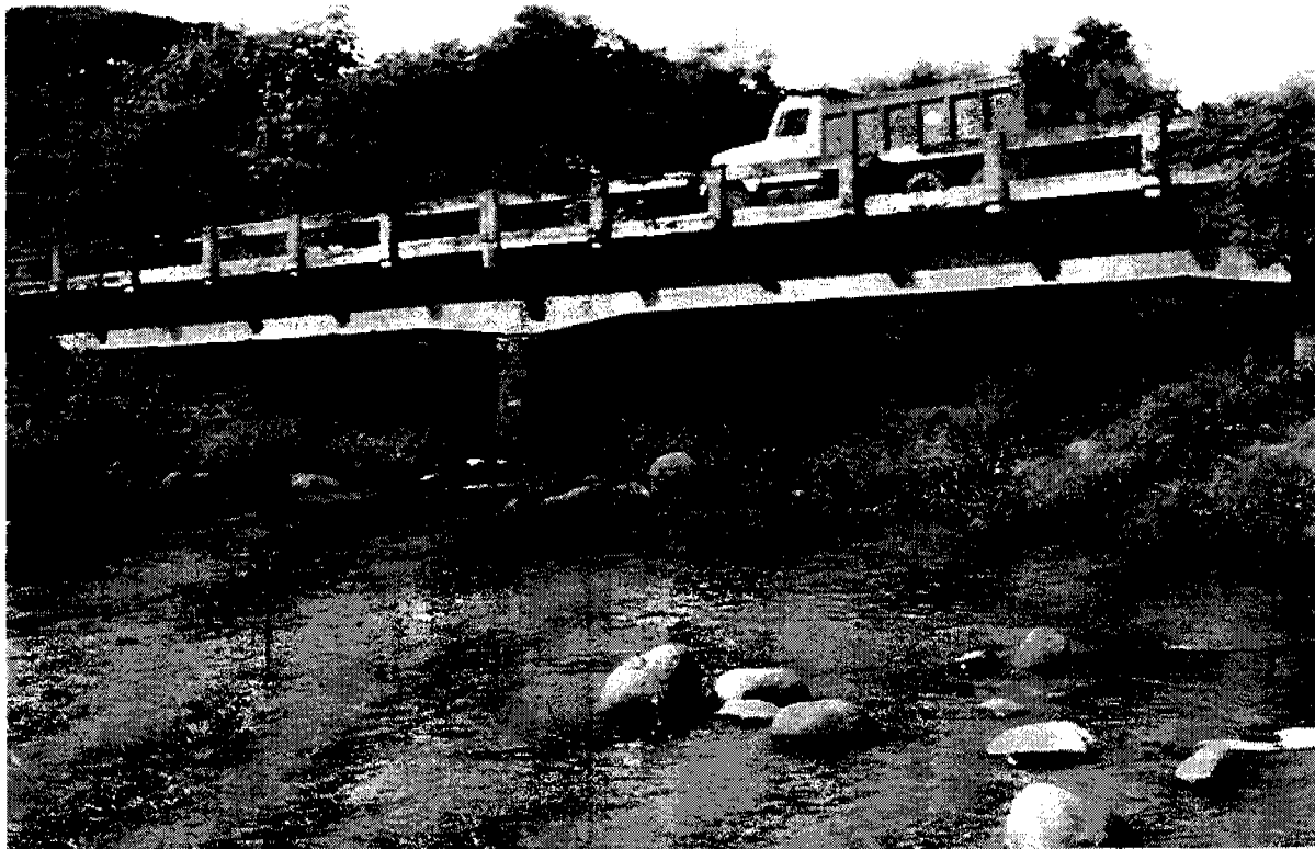
No. 6 The El Naranjo River. The bridge has two openings.
