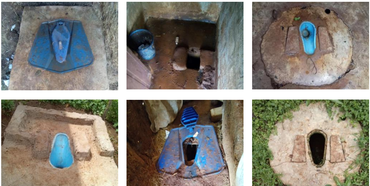
Figure 28: Examples of pit latrines defined as “improved” (i.e. with fully covered pits and floors around the drophole made of washable materials)
