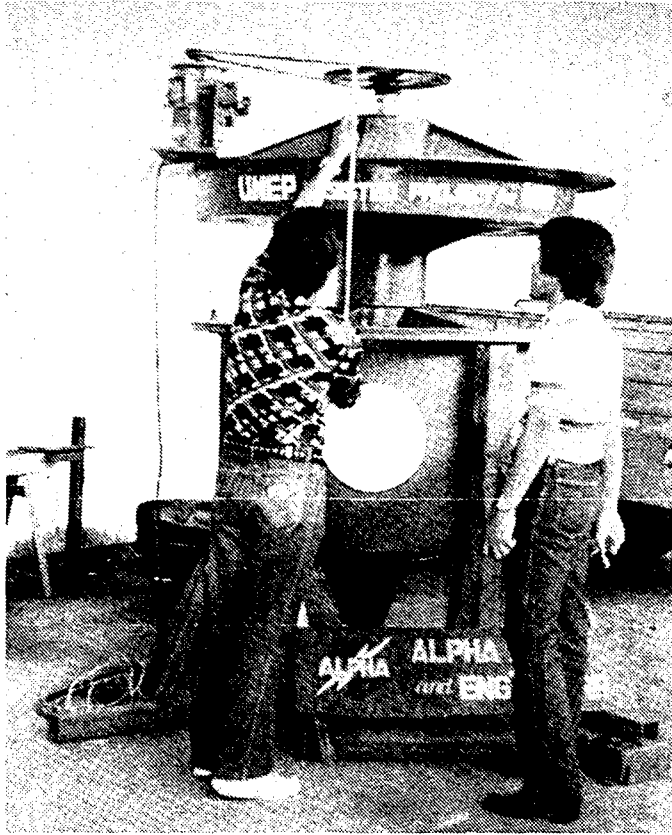
Fig. 7. Turbine-Runner Assembly
