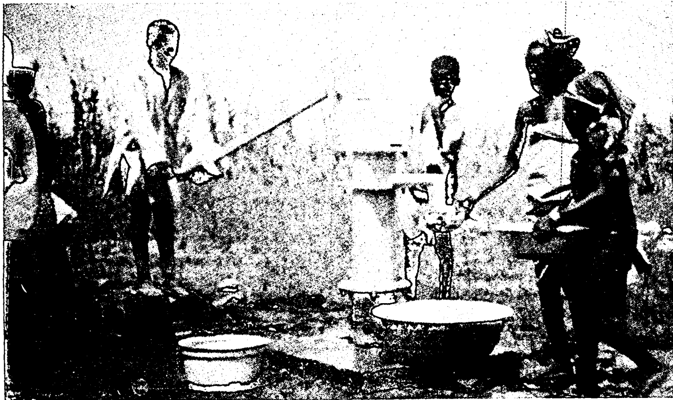
Extra Heavy Duty India Mark II Hand Pump designed to draw water from 85 metres, in operation in Sokoto, Nigeria
