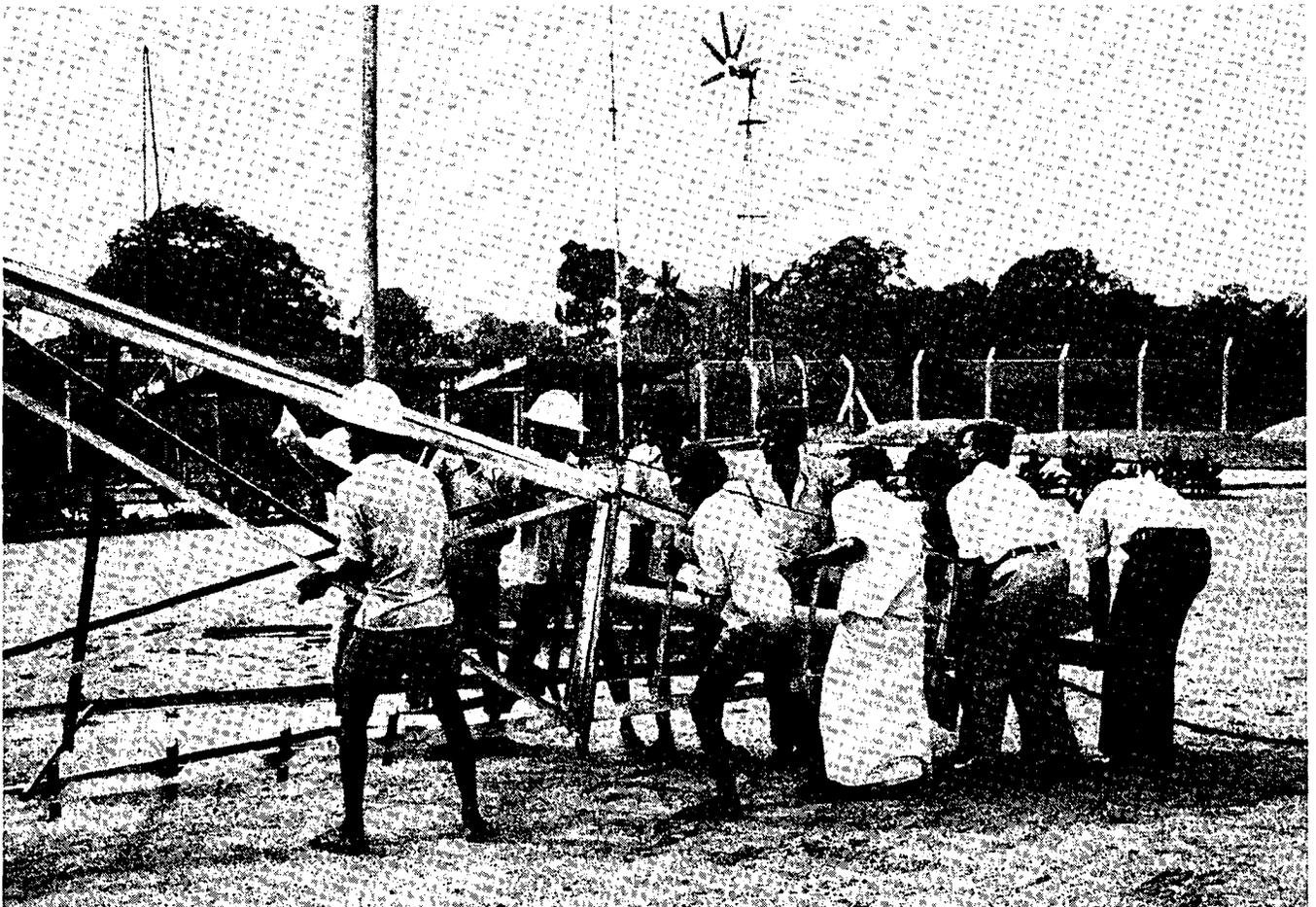
*The installation of a  $\varnothing$  5 m windmill in Colombo, Sri Lanka; in the background the  $\varnothing$  3 m WEU-I windmill.*
