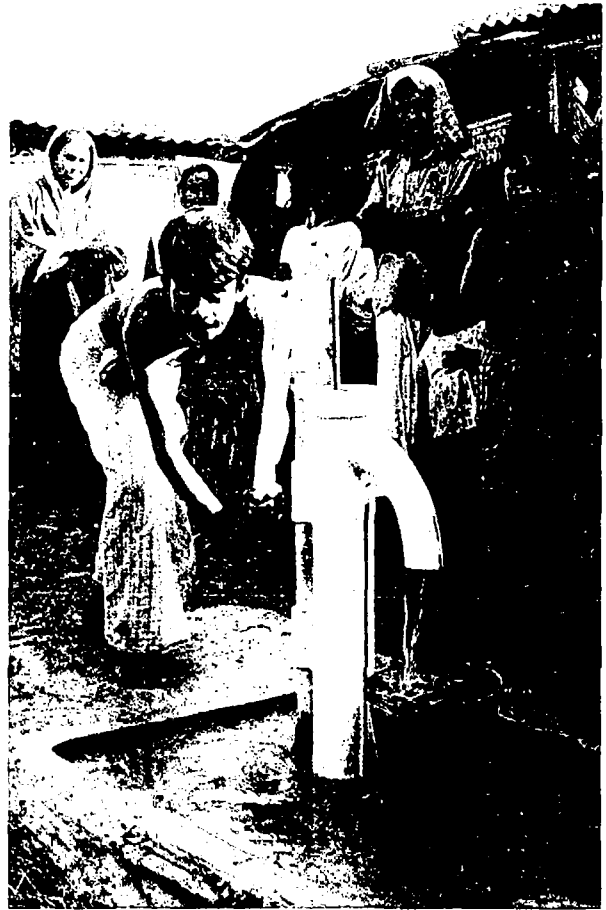
Pump No. 1 Installed
