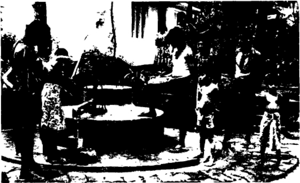
Fig. 1. View of well showing drainage channel to remove spilled water and stone layer to assist drainage
