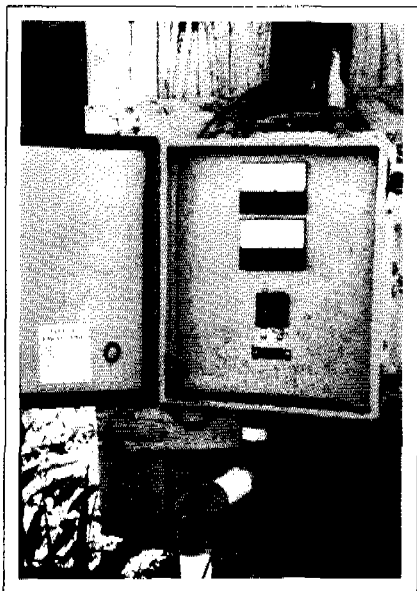
A solar pump control panel.
