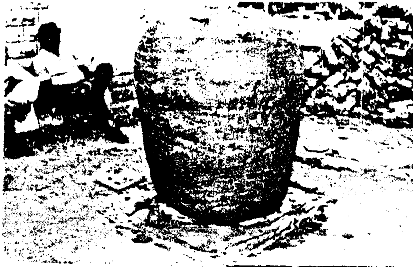
Fig. 16 - Mortar applied over the sack mould
