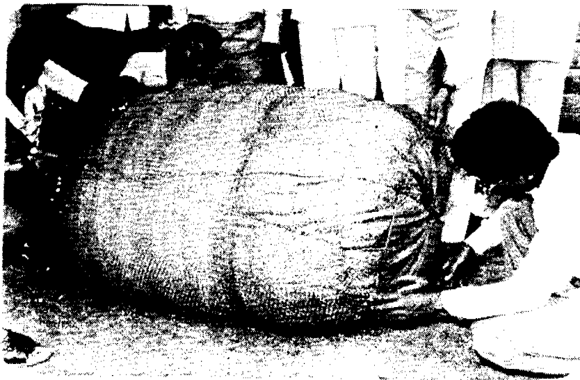
Fig. 15 - Sack Mould is filled with rice husk and reinforcement cage made over it
