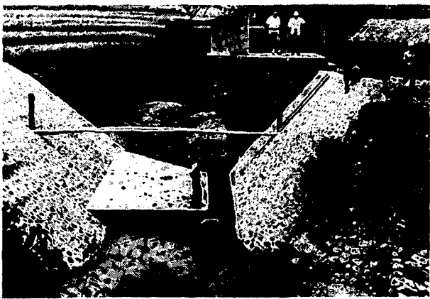
Figure 7. Artificial control to stabilize stream bed, steep gradient (Tributary of upper Solo River, Java, Indonesia).
