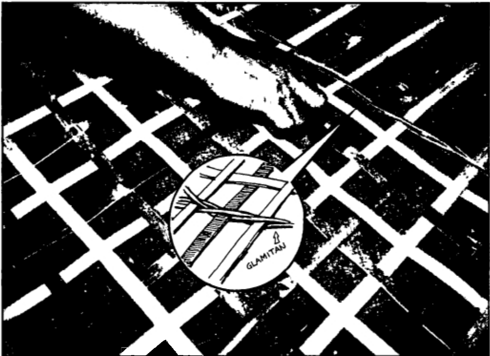
Bamboo twine holds the woven sheets together
