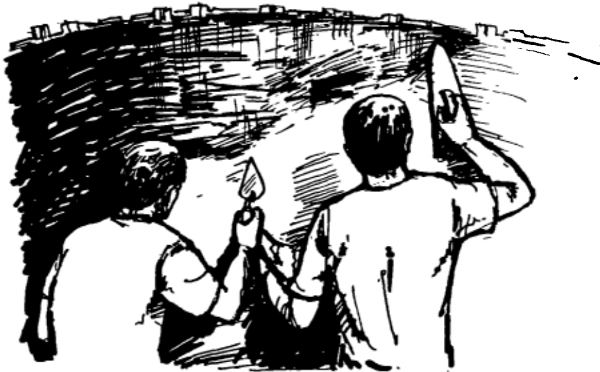
A second coat of plaster is applied with masonry trowels
