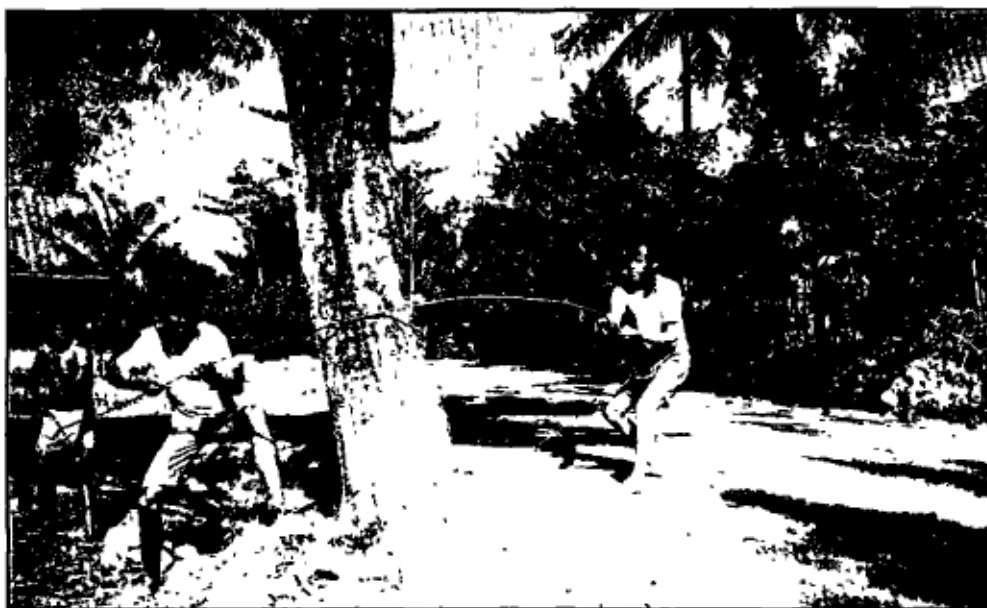
Bending rebar
