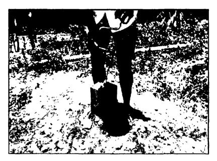
A post is buried to provide a support for the pivoting template and a hole is drilled . .
