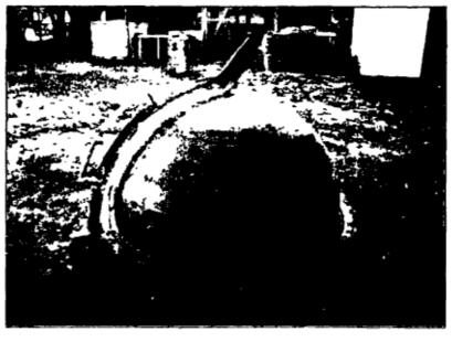
After smoothing with soil, sand and cement mixtures a cement and water 'slurry' was added . . .
