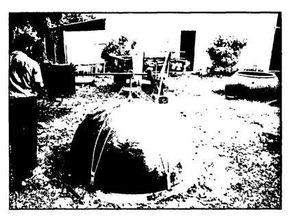
After at least one day of curing a special 'puller' is used to lift the casting a few inches from the mold.
