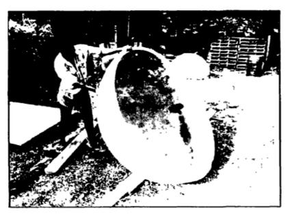
The castings are carried into position or rolled as shown. Or they could be joined first by tipping their mortar covered edges together and the sphere later rolled to the site.
