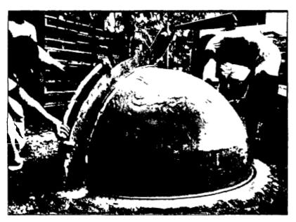
The following day a cement, water and fine sand mixture was used to finish the mold.
