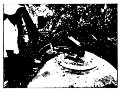
The upper half of the tank is cast in the same way. A lip can be shaped with a sheet metal template clamped to the pivoting template as shown.
