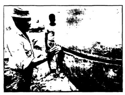
A rich cement and fine sand mortar is leveled into the groove. . .
