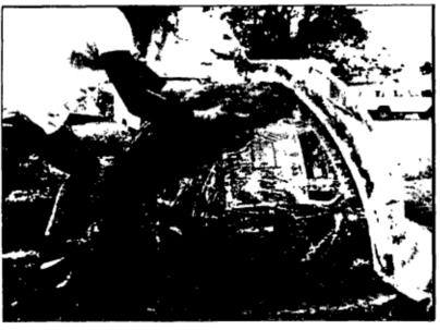
Cement mortar is then applied by hand using the pivoting template as a guide. Various mixtures were tried but 2:1 (sand: cement by weight) was used most often. Steel fibers (14.5mm or 0.57" straight lengths) were added for reinforcement.
