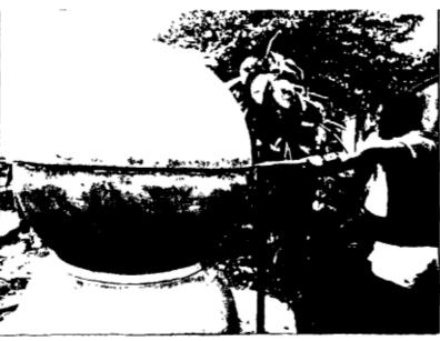
... and the top half is dropped one side at a time to join the castings. A cement slurry coating on the seam from the inside may be needed to complete the seal.
