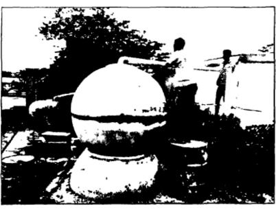
The tap is positioned to draw all of the water from the tank yet a bucket can still fit under it. A short stand pipe inside the tank (see the cross section, pg. 5) prevents sediments from being drawn out, but it can be lifted out for washouts.
