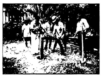
The template was found to be useful in aligning the post. If the axis is not exactly vertical it will not matter.
