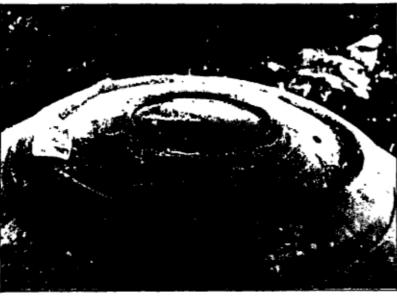
The lip provides extra strength and an accurate fit for the manhole cover / screened inlet cast in the position shown.
