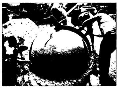
The casting was normally finished after a few hours (or the next day) with a mixture of plain mortar (no fibers) to bring the final thickness to about 20mm (3/4").
