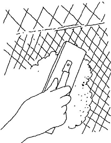
58. The mortar is applied by hand to the walls of the tank using a plasterer's steel float and builder's hawk. A layer of mortar not exceeding 15 mm is trowelled onto the formwork from the base of the tank upwards just covering the reinforcing wires. Continue on and around the tank, plastering on the first layer of mortar.
