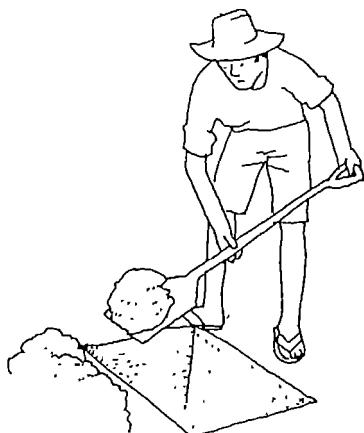
19. Having decided on the type and size of tank to be built and its proposed location in relation to the building, check that the sub-soil can support the weight of a full tank. By digging a small trial hole it can be seen if the ground is soft or swampy. If the ground is unstable, a lot of work will have to be done to build and ensure a strong foundation and base for the tank
