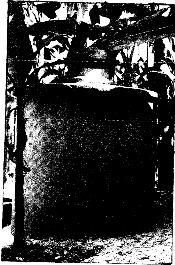
Figure 6. Bamboocement RWC volume 2\frac{1}{2} m 3
