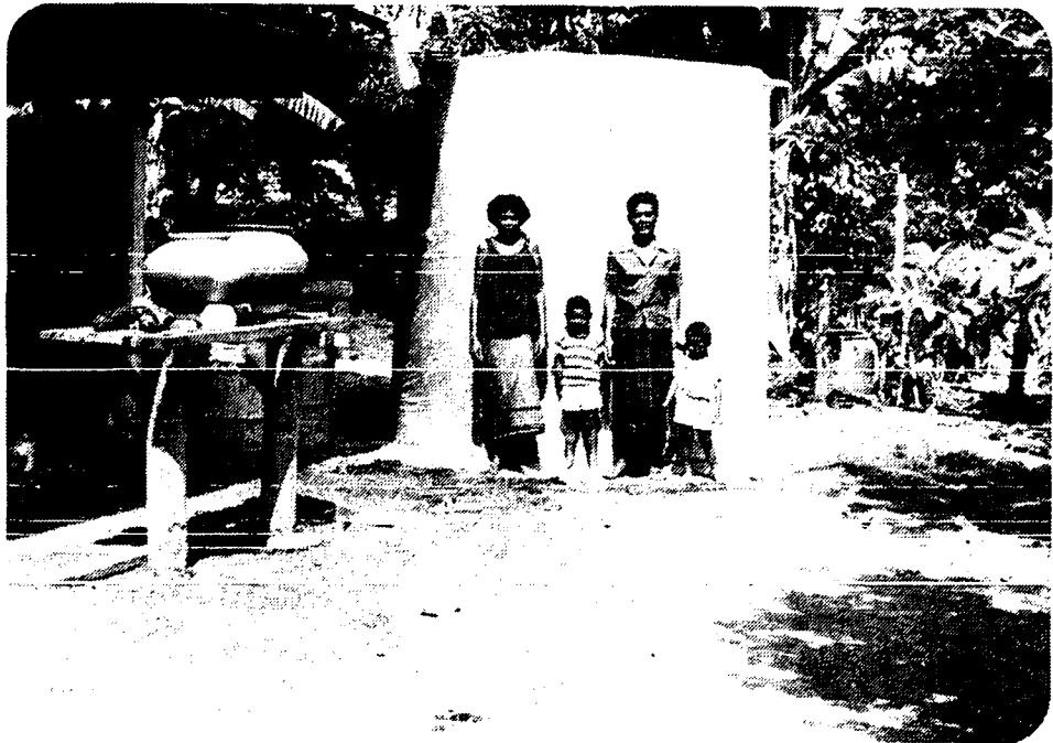
Figure 8. Water tank is being cured in PVC sheet.
