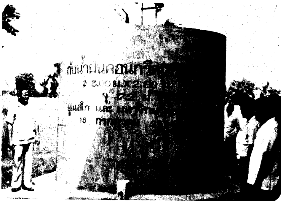
Figure 5. A demonstration tank
