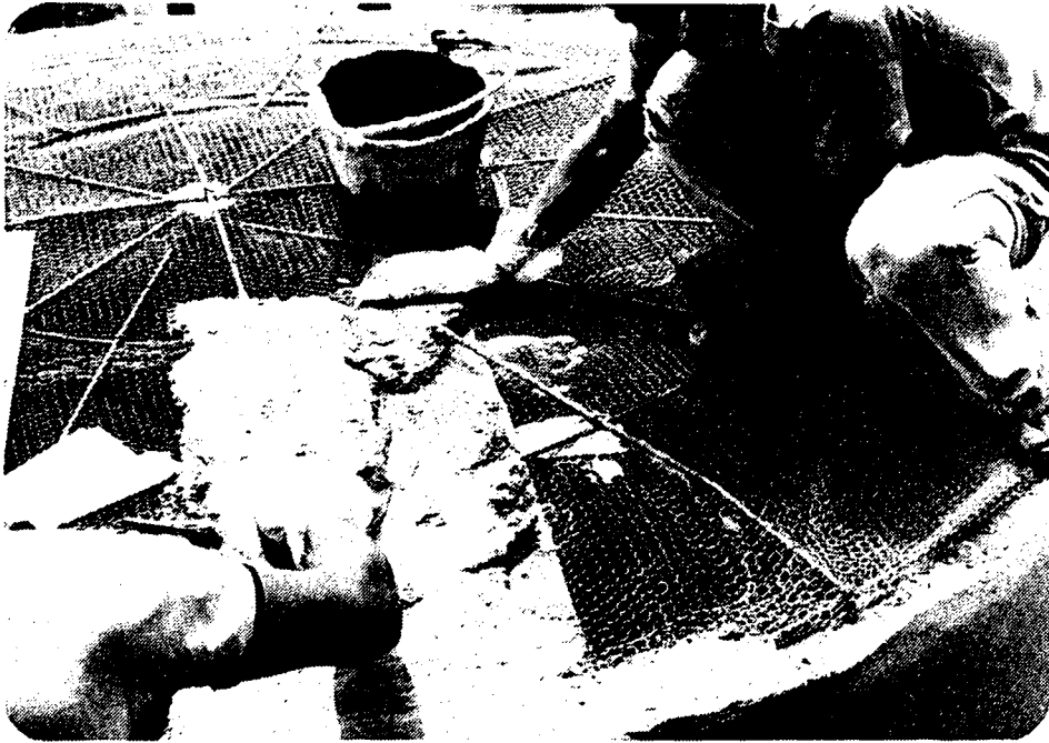
Figure 8. Plastering of roof
