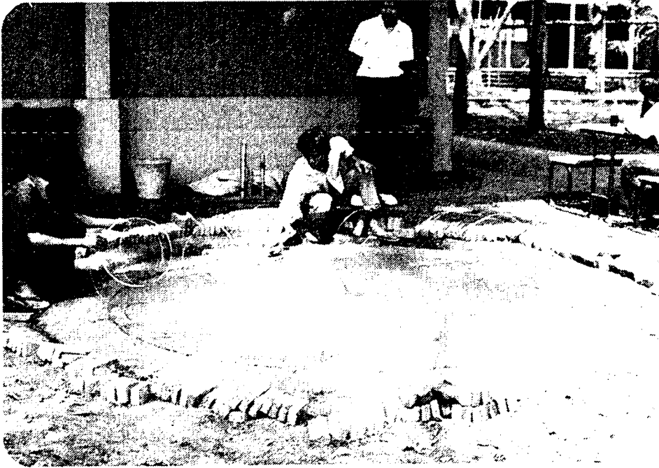
Figure 4. Construction of base
