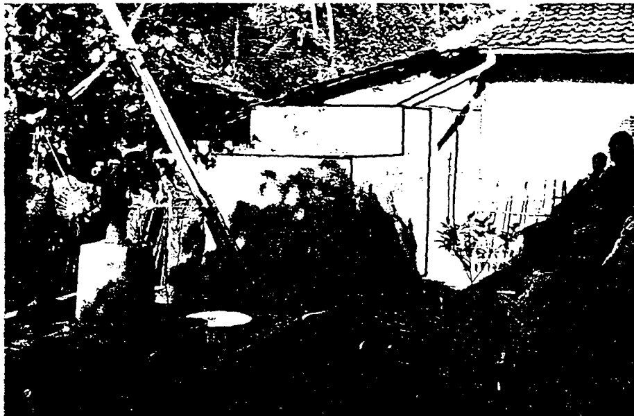
Figure 5 Reinforced concrete RWC volume 10 m 3 in desa Tanjakan. With handpump made in Central Java
