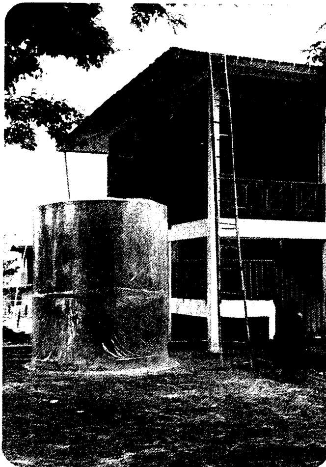
Figure 9. Curing of water tank
