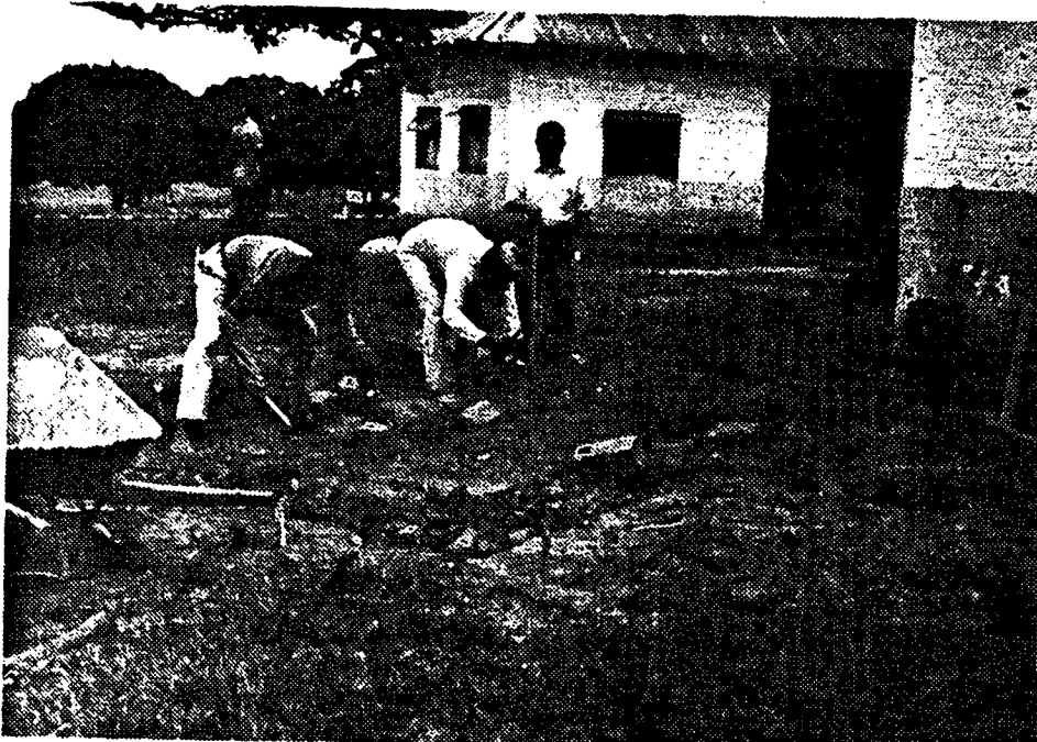
Starting footings for hospital tank.
