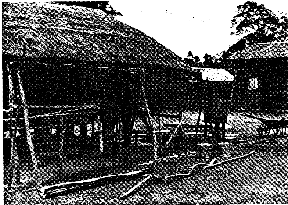
Finished thatch roof RWS system.
