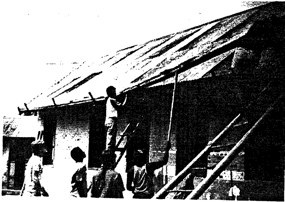
Intstalling gutters.
