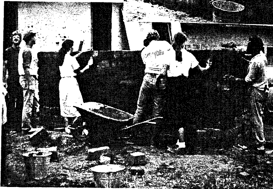
Cementing tank walls.
