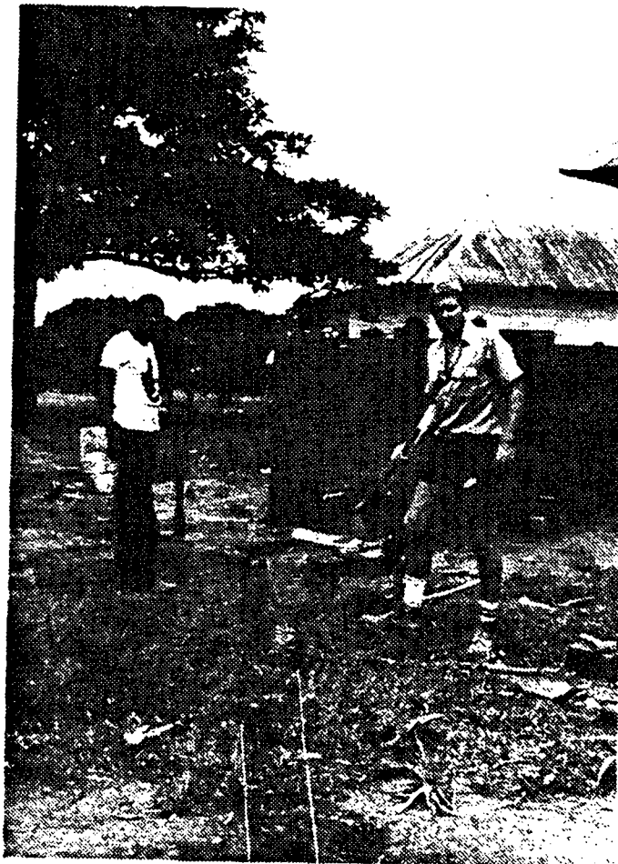
Digging evacuation channel.
