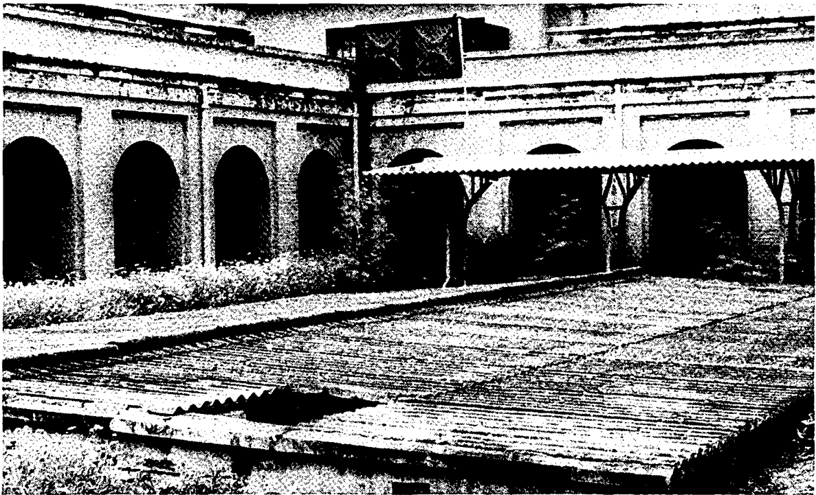
Rain water collection tank with provision for pump-set installation, including overhead tank for distribution to laboratory
