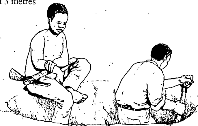
Community participation in Well Digging
