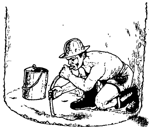
Removing water from the cutter holes
