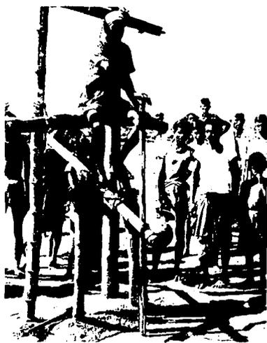
Fig. 5.7 **BAMBOO SCAFFOLDING, PIVOT AND LEVER USED IN DRILLING BY THE SLUDGER METHOD.** (From "Jetting Small Tubewells By Hand," *Water Supply and Sanitation in Developing Countries*, AID-UNC/IPSED Item No. 15, June 1967.)
