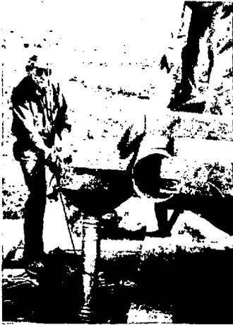
Fig. 5.37 PLACING GRAVEL-PACK MATERIAL THROUGH PIPE USED AS TREMIE.
