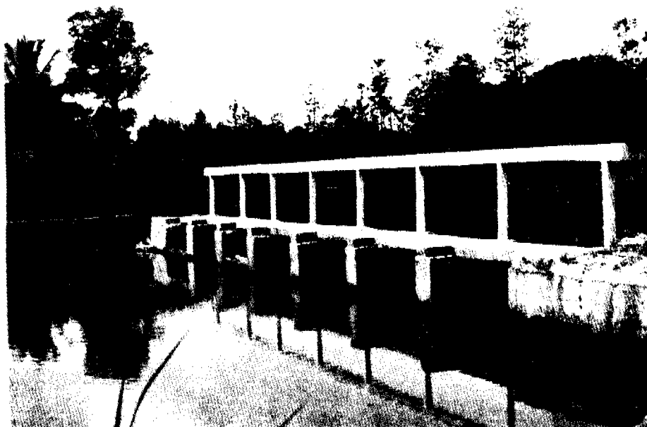
Fig. 2. Upstream view of the small weir in Ubon Ratchatani province, built under the People's Volunteer Weir Program
