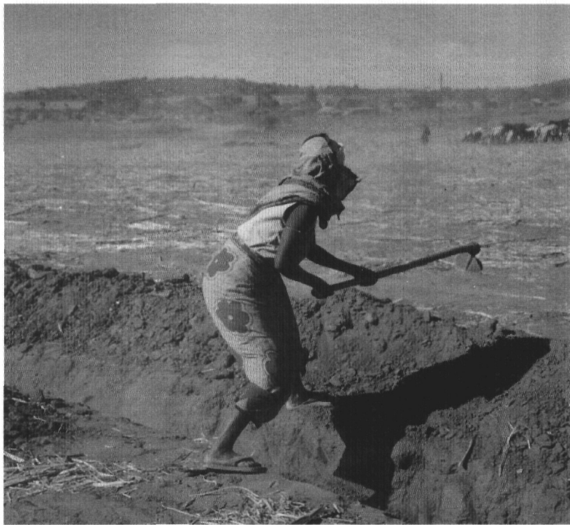
A woman in Njoro village works to install a pipeline through an agricultural area.
