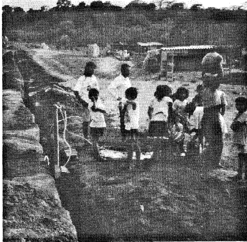
Community built water line in El Salvador.
