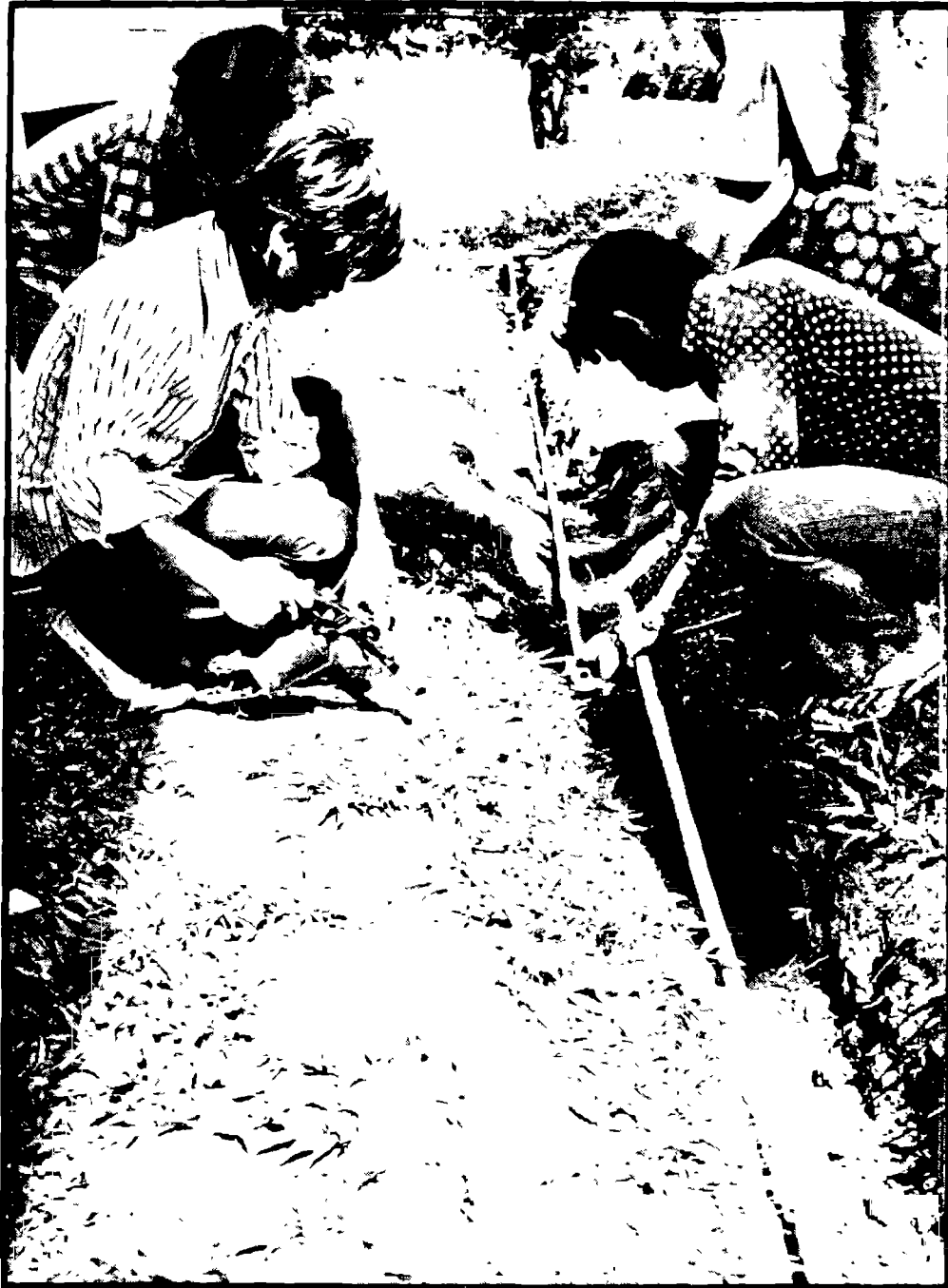
Illus. 12. A gravity system being installed. (Source: WHO, Photo by J. Abcede.)
