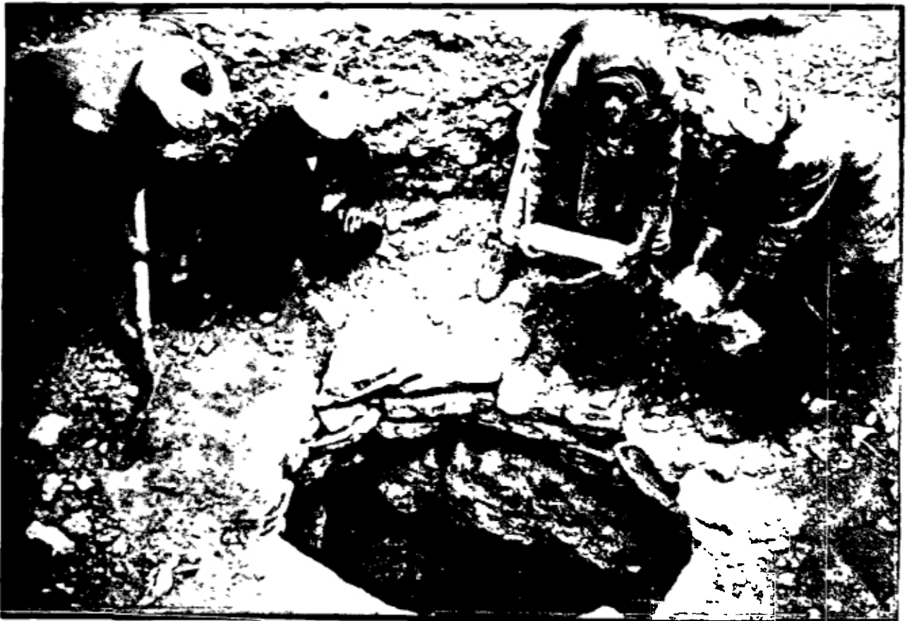
Illus. 18. An open dug well subject to contamination. (Source: UNICEF.)
