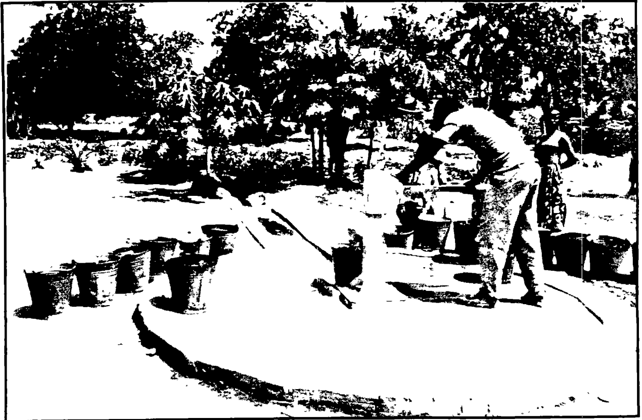
Illus. 6. A protected well. (Source: Bob Blankwaardt, Hand Drilled Wells: A Manual on Siting, Design, Construction and Maintenance . Rwegarulila Water Resources Institute, Dar Es Salaam, Tanzania, 1984.)
