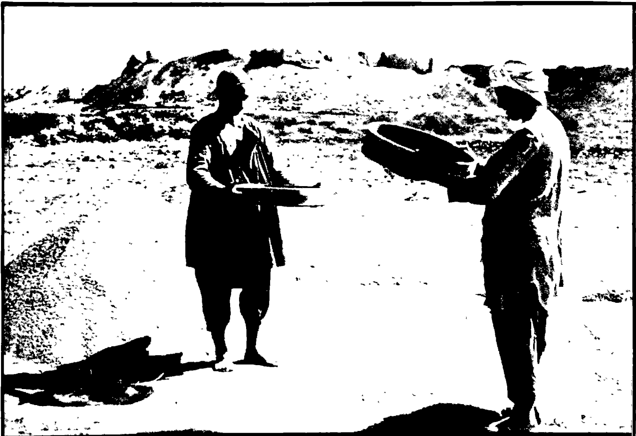
Illus. 4. Sand gathered by villagers for mixing concrete. (Source: UNICEF.)
