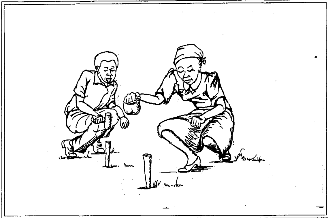
5. Pegging of latrine
