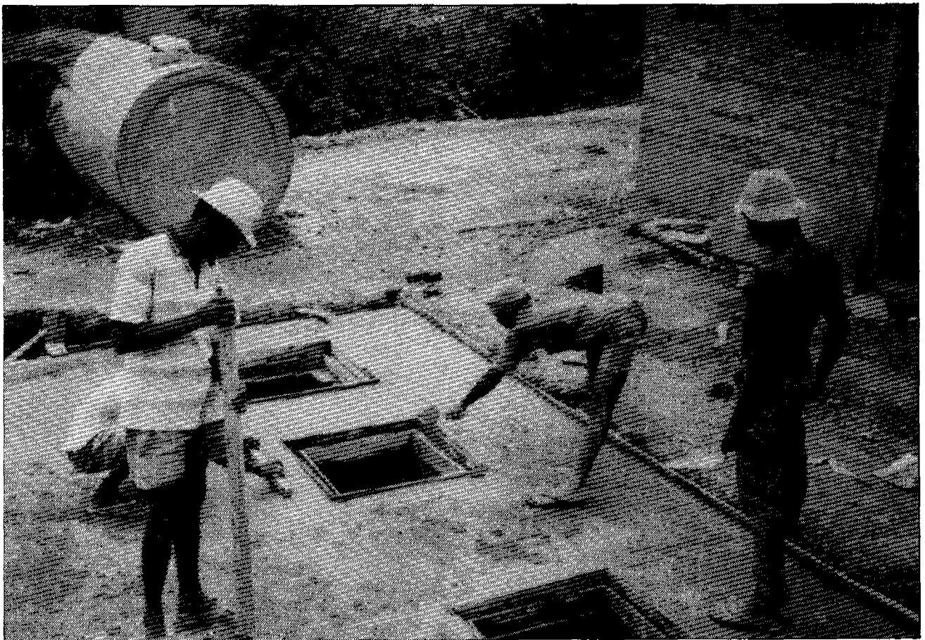
Figure 7. Construction of septic tank through community construction contract
