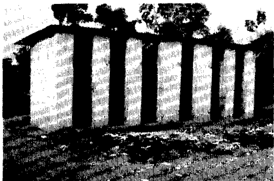
Many schools have latrines that have fallen into disrepair. (Togo)
