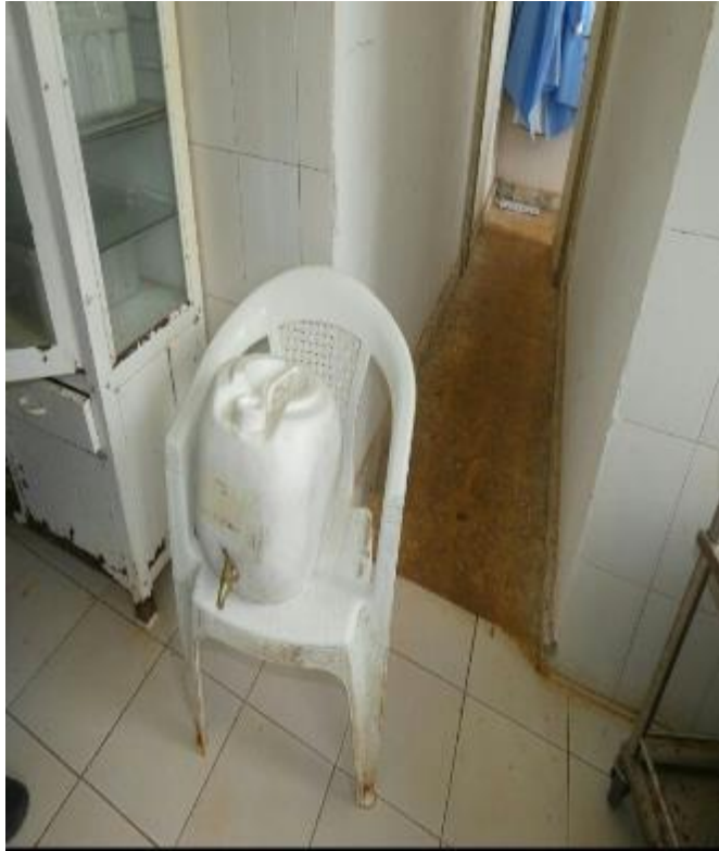
Hand washing station before CCM, Wetet Abay HC/Photo CRS staff
