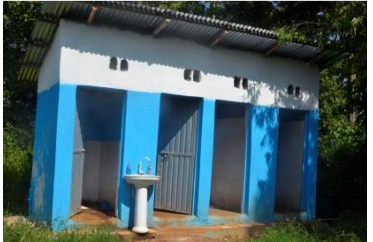
Staff toilets after CCM, Wetet Abay HC/Photot CRS staff
