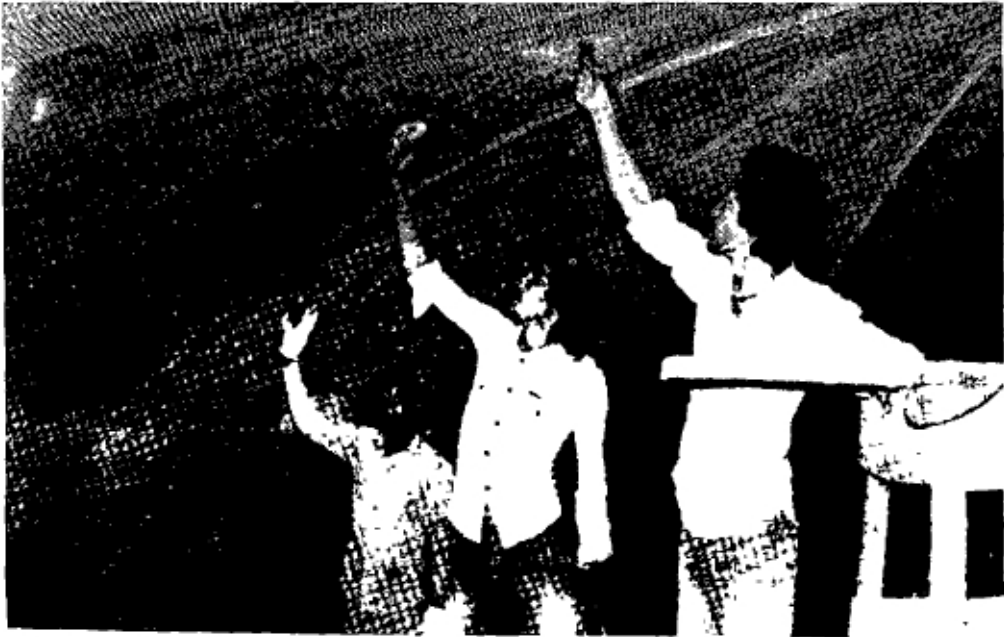
Fig. 59 Plastering ferrocement ceiling dome
