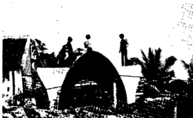
Fig. 22 Ferrocement gothic vault shelter
