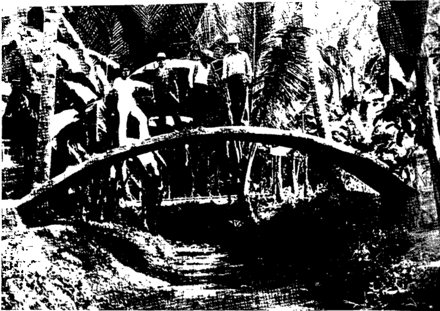
Fig. 7 (Ferrombo) of bridge: Bamboo reinforced combined with chicken wire span 7.8 m: 1.5 m width: curved shape prevents damage from flood.
