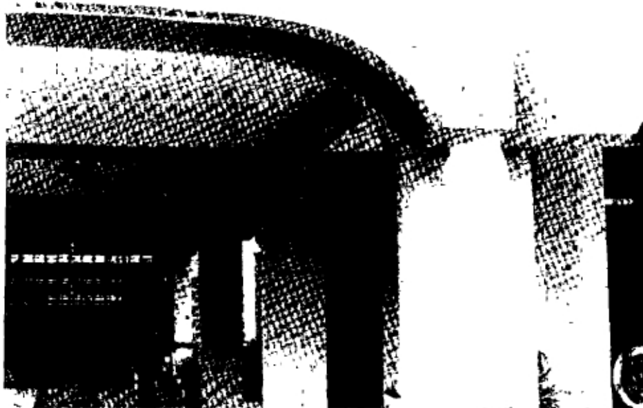
Fig. 78 Typical rib structure of ferrocement canopy
