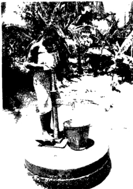
Figure 5.1. NIRA AF-85 direct action pump (Photo J. Viiala).
