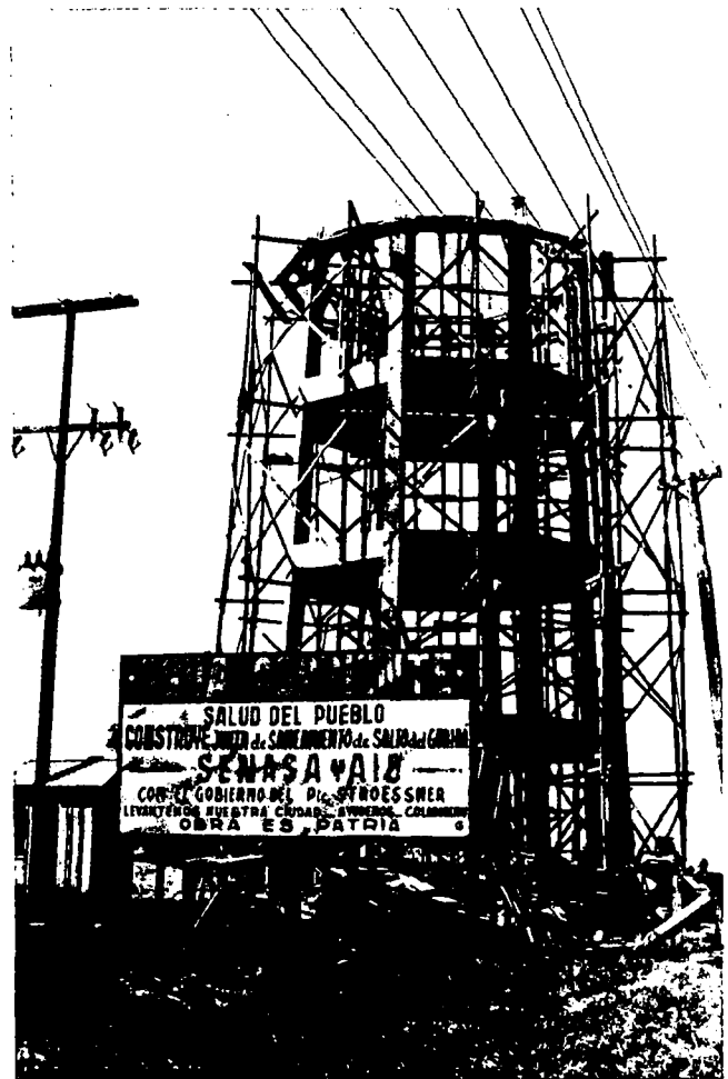
Construction of a large community storage tank is one means of water storage.
