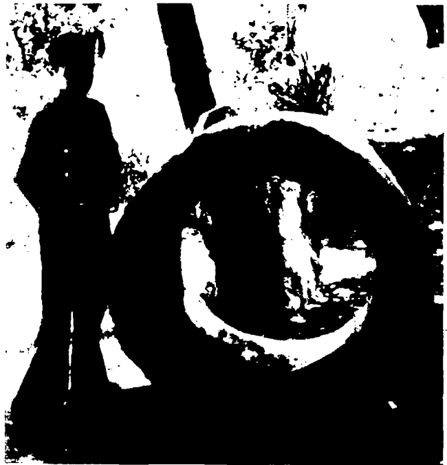
Rings to cap wells and other parts of water supply systems may be constructed locally.
