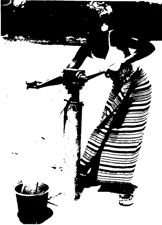
Appropriate technology using simple systems such as this hand pump is usually a better choice in rural areas than more advanced technology.
