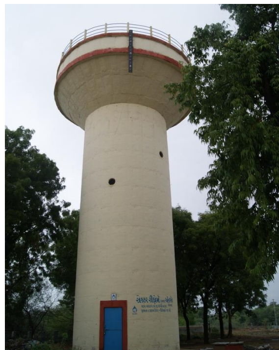
Photograph: Infrastructure built from the 90-10% contribution
