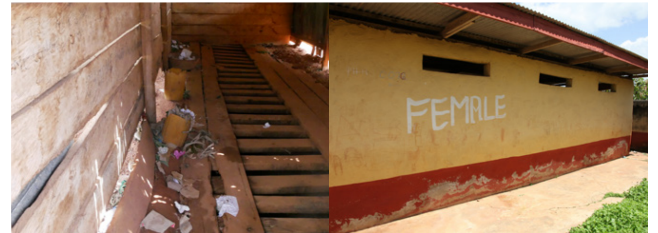
Inside an unimproved public toilet in Asamang (left) and a public shared toilet showing the female side (right)
